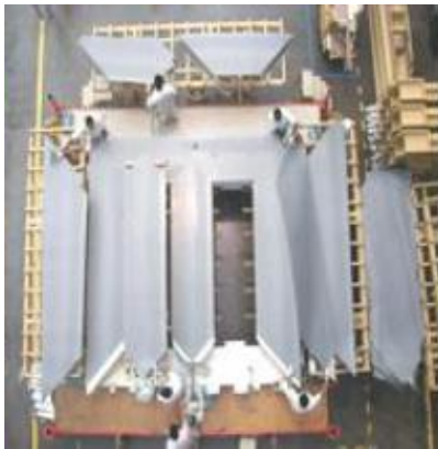
Fig. 1. Stacking of transformer core plates in step-lap.
